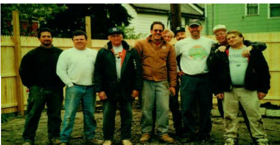
Below, with Mike Renzi and a men’s group from Rochester, building the fence around “Grace House.”
